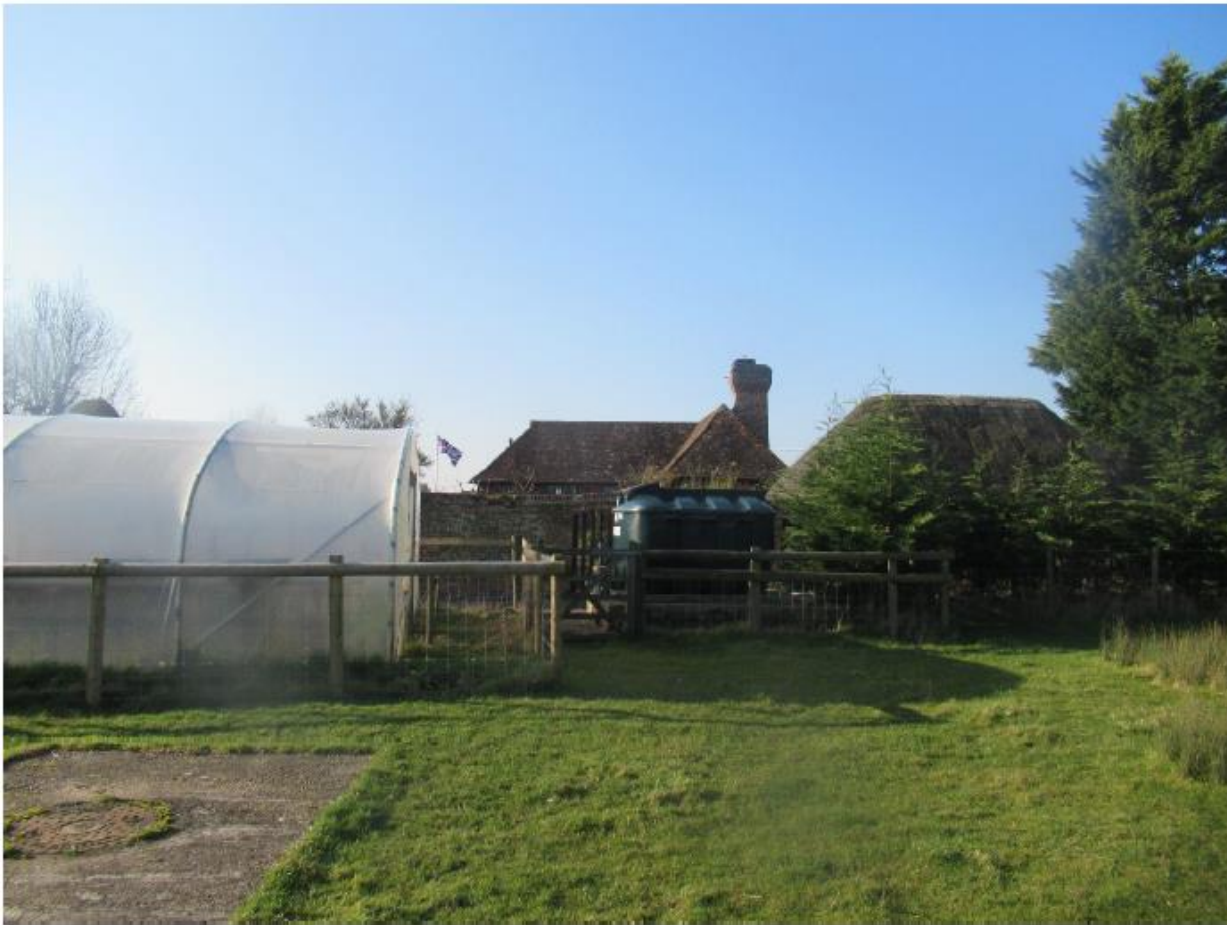
Figure 6.1: View towards Northern Elevation of Stonelees (Grade II* Listed Building)
